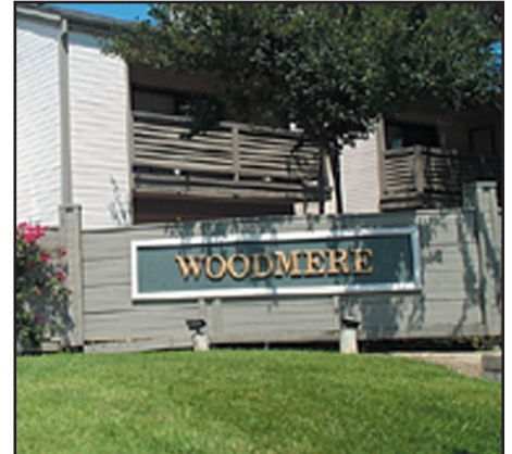
Woodmere Apartments, at 910 W. Phillips St., Ontario, is one of the many apartment complexes Mogharebi sold last year.
