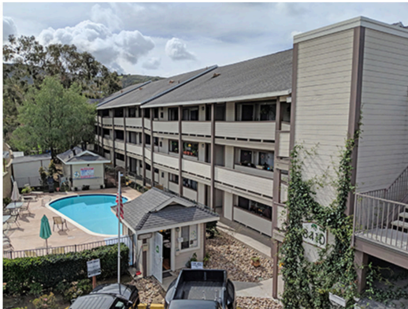
Willow Creek in El Cajon, Calif., features 33 apartments, a swimming pool, covering parking and hillside views.
